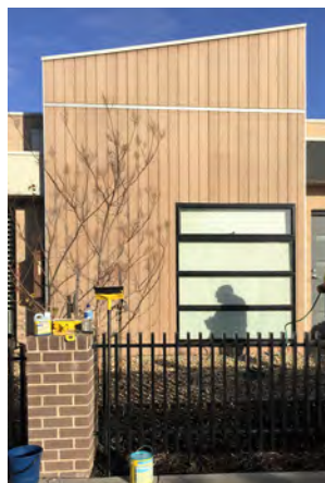
36 MONTHS: The boards are now very light, and are about to begin to be restored.
