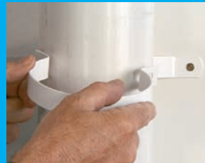
Step 3 – Place pipe into bracket base.
