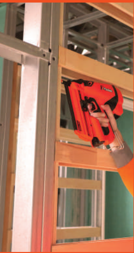
Steel Frame Fix out
