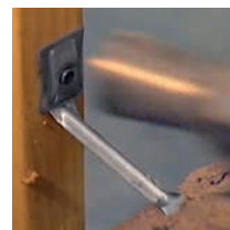
Hammer vibration can loosen the connection of ties to the mortar
