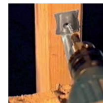
Screw ties directly to the frame for both face fix or side fix ties
